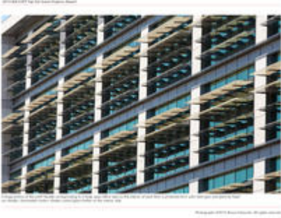
Automated window shades control glare on the south facade of the building - Photo Credit: Photographs ©2012 Bruce Damonte. All rights reserved.
