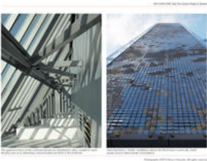
View of the uppermost floors of the northwest facade chamfered to allow sunlight to reach play area of elementary school to the northwest & view of Artist Ned Kah's "Firefly" installation that adorns the Wind Tower's north side. - Photo Credit: Photographs ©2012 Bruce Damonte. All rights reserved.
