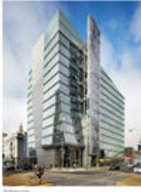
Northeast corner of SFPUC - Photo Credit: Photographs ©2012 Bruce Damonte. All rights reserved.
