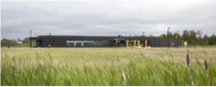
Reconstructed Wetland - Photo Credit: Frank Ooms
