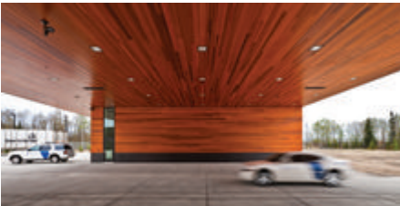
Primary Inspection Canopy - Photo Credit: Paul Crosby
