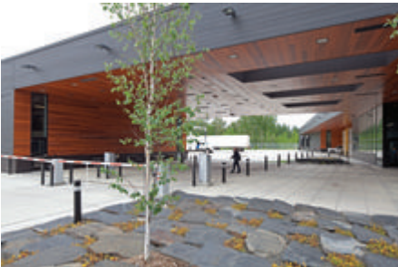
Secondary Inspection Canopy - Photo Credit: Frank Ooms
