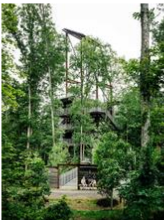
Phototropic structural frame elevates renewable energy elements above the forest canopy. - Photo Credit: Photography by Joe Fletcher
