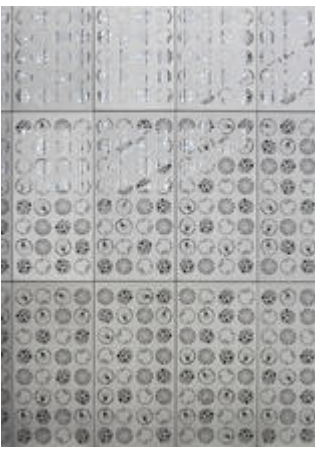
Stainless steel wall panels with magnified cutout images of local photoplankton - Photo Credit: Photo by Bruce Damonte
