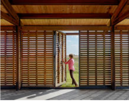
The sliding, wood slat doors also have operable panels. - Photo Credit: Casey Dunn
