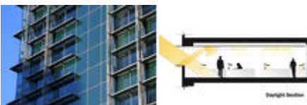
Because of the importance daylighting plays in human health and comfort, the project optimized daylighting in the perimeter zone utilizing a task/ambient approach to lighting. - Photo Credit: SERA
